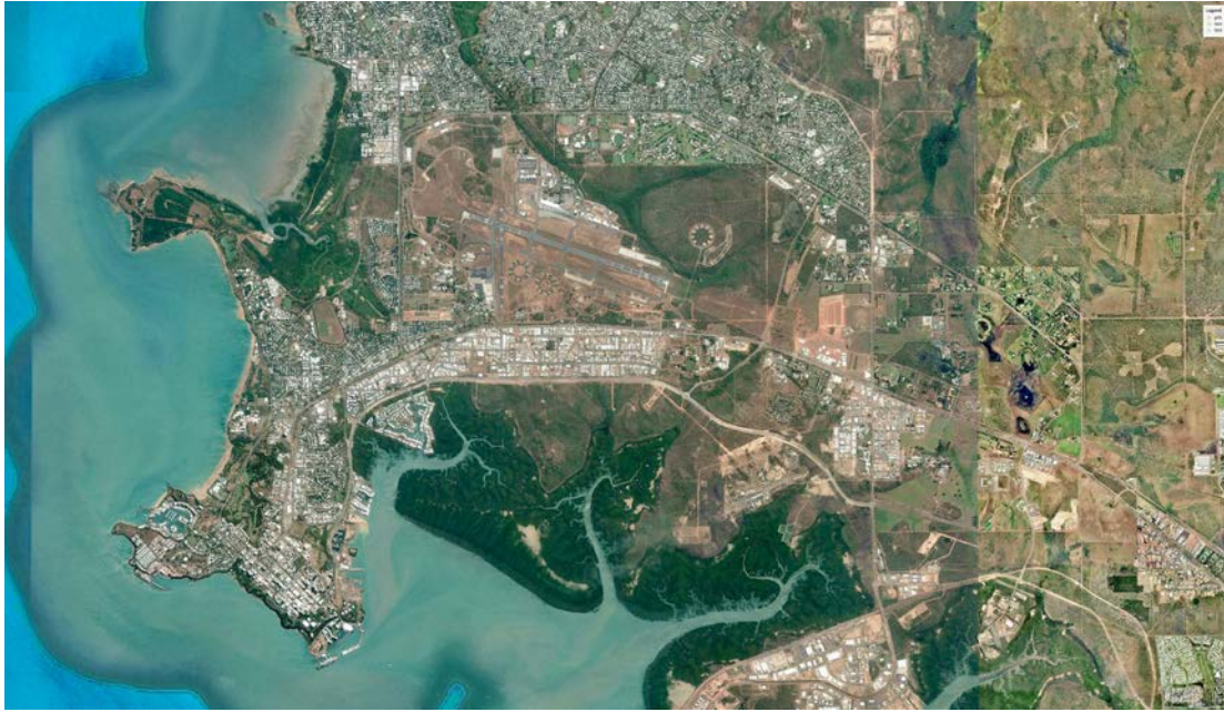
Figure 2: Aerial photograph of Darwin
